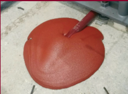
Chockfast Red HF being Pumped
