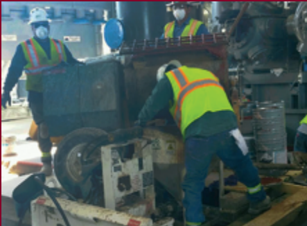
Mixing Chockfast Red HF
